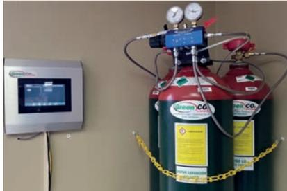
© Green CO<sub>2</sub> Systems | Left. Green CO<sub>2</sub>'s Green Touch Controller is a specially designed leak detector with flow control and automatic shutoff capabilities. | Right. Green CO<sub>2</sub> Systems Founders (l to r) Dan Schneider, Mike Schutte and Brett Schutte.
